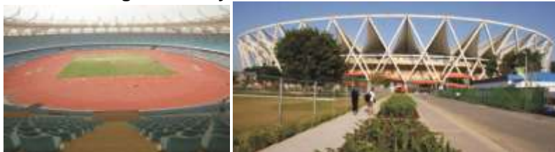
Outside view of J.N. Stadium Inside view of J.N. Stadium
