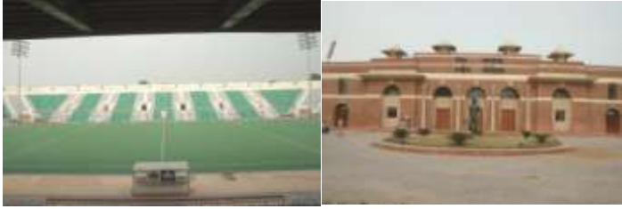
Outside view of Major Dhyan Chand National Stadium Inside view of Major Dhyan Chand National Stadium
